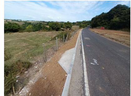
Dover Road, Phase 1 works crossing
