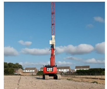
Band drain installation
