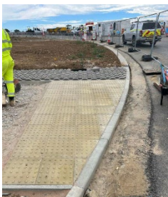
Installation of Tactile Paving with Pedestrian deterrent paving
