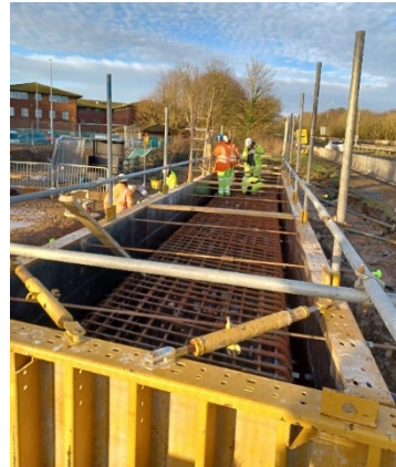
Reinforcement and Formwork
