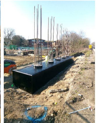
Protective coating added
