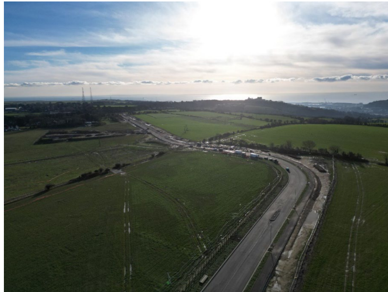
Looking across Section 2 - January 2023
