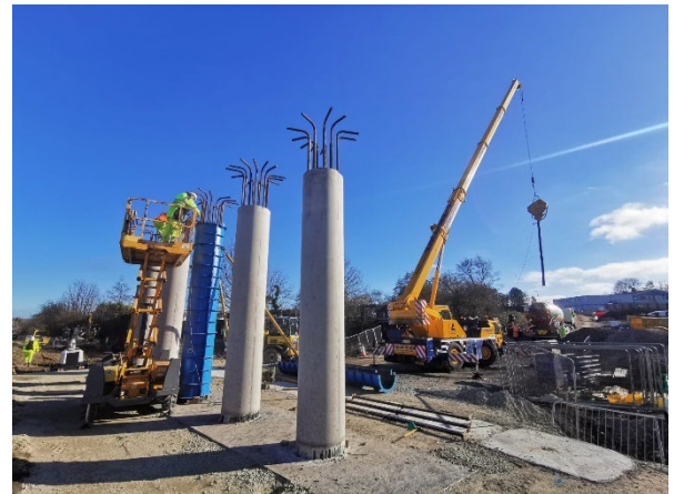
Column Installation - Section 1b South
