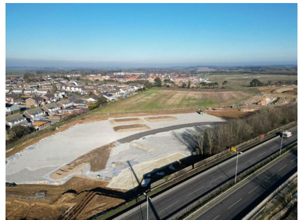
Construction of the trial embankments and temporary access road for the piling works - Section 1b North
