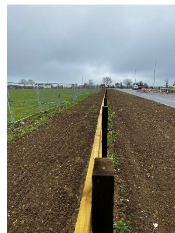
Section 2 landscaping and fencing installation.
