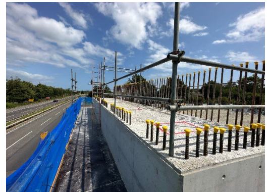
Image: Crosshead in Section 1B south
