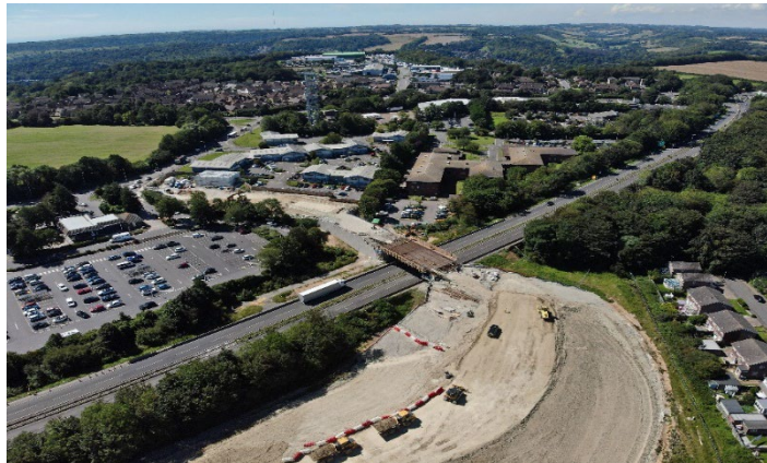
Image left shows Drone image above new bridge.
