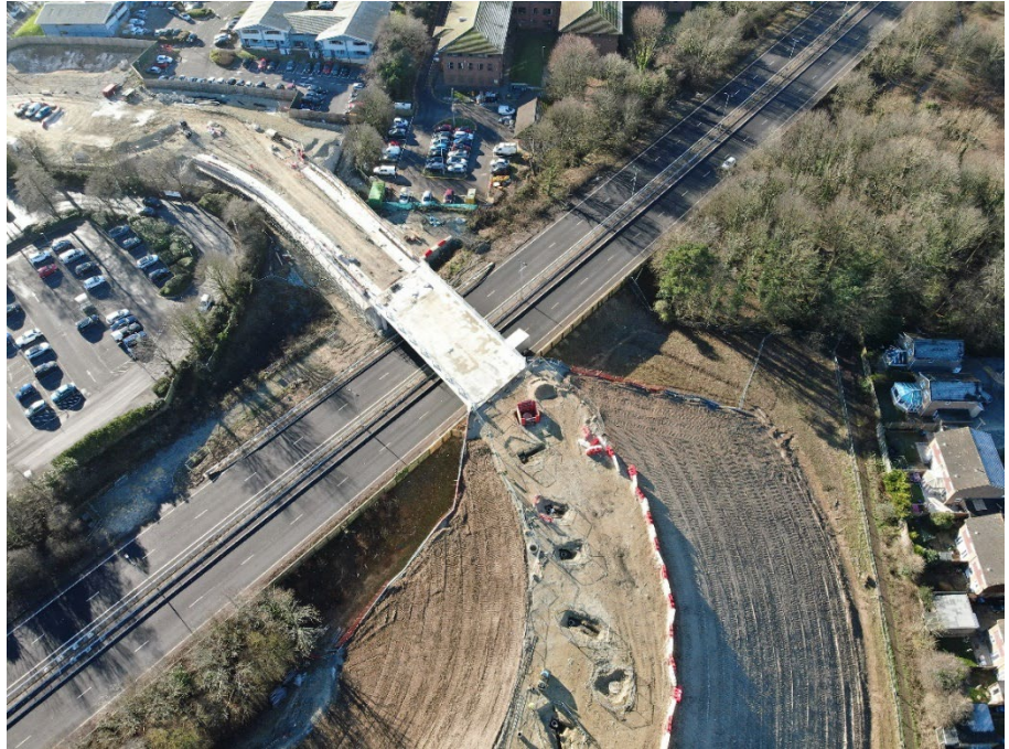
Image above shows Section 1b North (new bridge and embankment) and construction of gullies.
