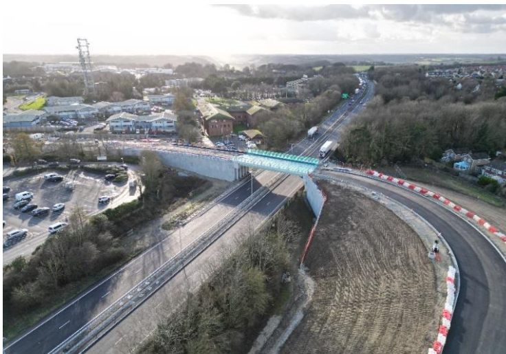
Image above shows Section 1b North (new bridge and embankment) and construction of asphalt.
