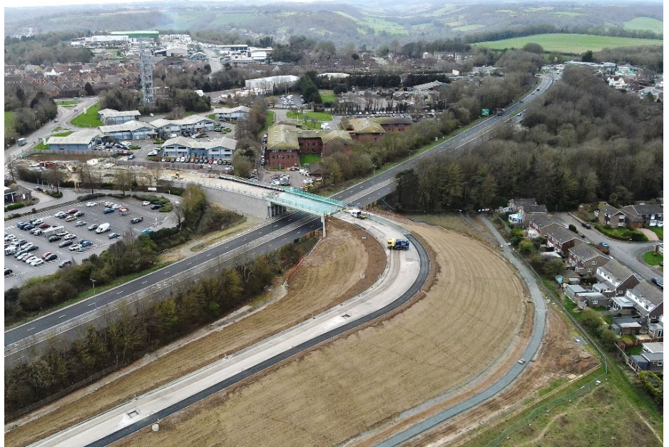
Image above shows Section 1b North (new bridge and embankment) and construction of asphalt.
