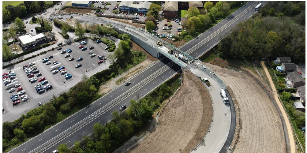
Image above shows Sections 1B North (new bridge and embankment) and 1B South (towards Tesco roundabout) and construction of asphalt.
